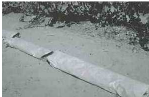
Figure 2-4. Types of rolls from left to right: biscuit, cigarette, and flop.
