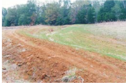
A newly installed terrace to slow water runoff.
