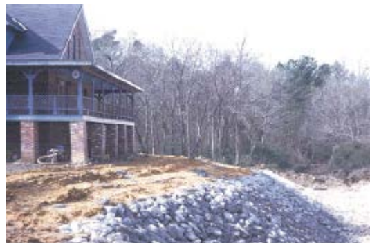
Rocks placed along a streambank to control soil erosion.
