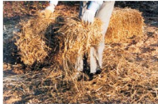
Covering newly prepared lawn with straw to control erosion.
