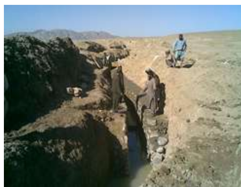
Karez canals require maintenance (Photo http://www.afghanistan.gc.ca )
