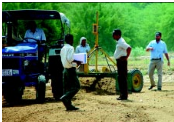
Fig.6. Laser leveler attached to a 4-wheel tractor.
