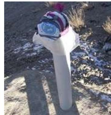
**Figure 15.** For curing, cover both pipes to reduce air movement. (Source: CRS, 2013).
