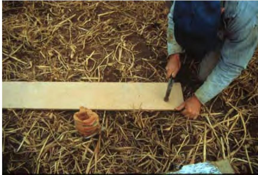
**13.) From the back side, drive approximately 24+ finishing nails (1" length) through the board being careful to stay more than 1" from the sides and about 2" from the top and bottom of the mount area.**
