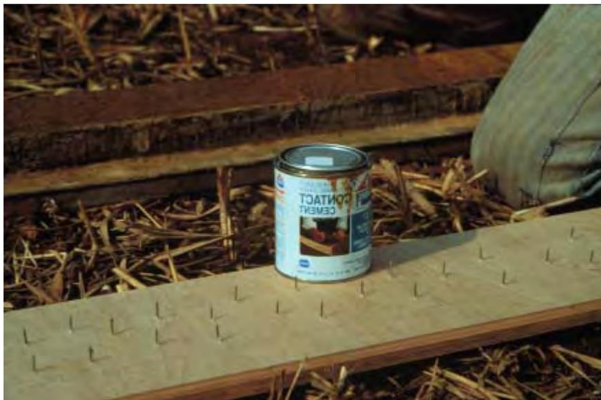
**14.) Apply a generous coat of Elmer's Contact Cement to the mounting board and protruding nails.**
