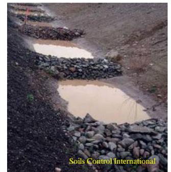
*Water trapped behind check dams will either enter the soil or evaporate. Note the accumulation of finer soil behind the dams, which would have washed away without the dams.*
