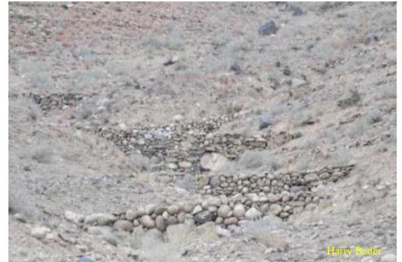
*Check dams can be constructed with local materials. This image shows roughly built check dams, which require little labor and maintenance. .*
